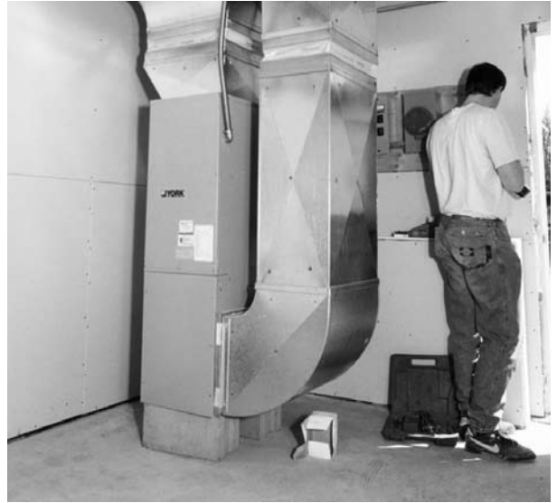
Air-to-air heat pump – interior unit.
