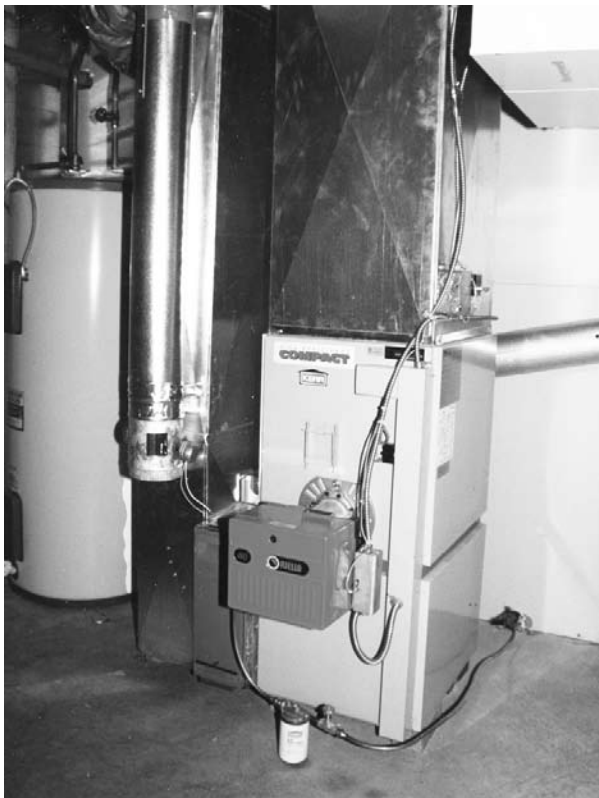
Modern warm-air oil-fired furnace.
