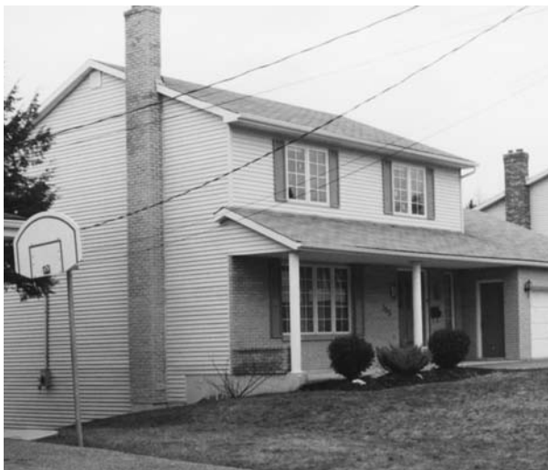
Establishing good draft can be very difficult in an uninsulated exterior chimney.
