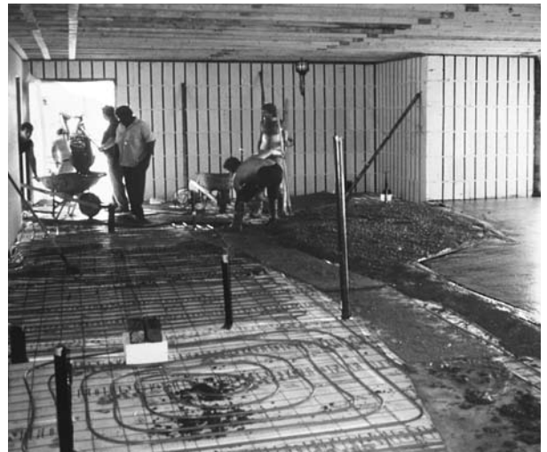
Placement of concrete floor slab on top of radiant floor piping.
