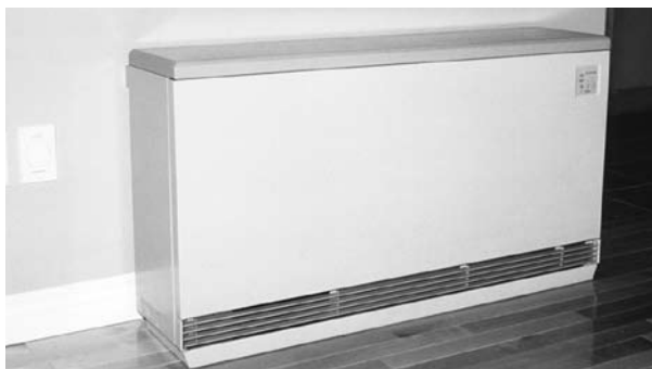
Electric thermal storage heater.
